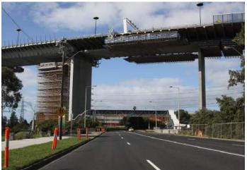
The West Gate Bridge Strengthening Project located in Melbourne is drawing to a close. Having worked closely with Australian construction company John Holland over the last 24 months, APS have supplied the suspended access platforms used to carry out the external concrete and steel strengthening works.
